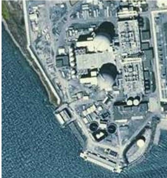
An overhead photograph of the southern New Jersey Salem I and Salem II reactors (www.maptech.com)
